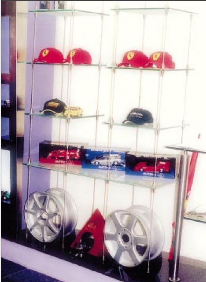
**Above:** A pair of sleek looking stainless steel suspended merchandising fixtures with shelves made of 12 mm glass. Stainless steel cables at the corners of the shelves appear to run the full length from ceiling to the floor. The top and bottom cables are anchored at respective ends in the ceiling and the floor.
