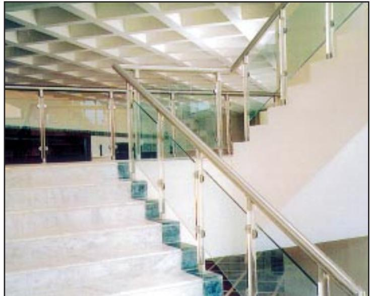
*Stainless steel handrails in combination with acrylic balusters and glass guardrails. The stainless steel clamps were specially designed to weld the top rail to the balusters and the baluster to the base plate at each step. The clamps are forged and machined to perfection and are designed as a two-piece system whereby the glass can be replaced without removing the clamps from the balusters.*
