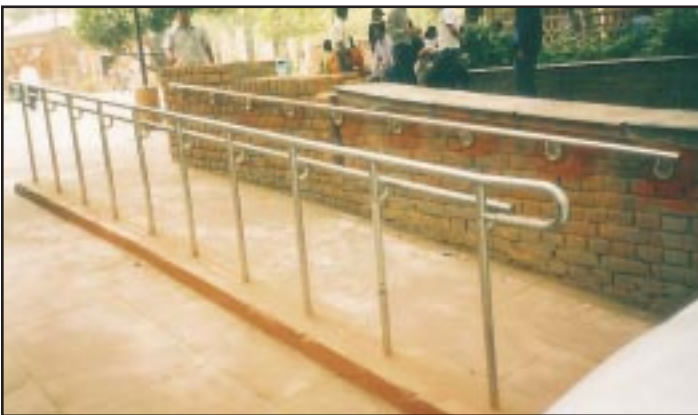
About 1,155 kg of stainless steel 316L tubes in brush finish have been used for making double-handrails at Delhi's 'Dilli Haat Food & Craft Bazaar', for the benefit of physically handicapped visitors. These handrails have been installed on sloping ramps; a total of 28 such ramps can be found at the bazaar, the length of ramps varying from 3 metres to 21 metres.
