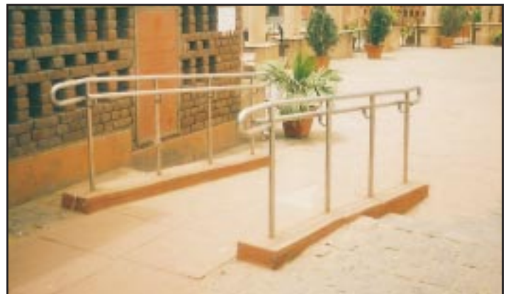
About 1,155 kg of stainless steel 316L tubes in brush finish have been used for making double-handrails at Delhi's 'Dilli Haat Food & Craft Bazaar', for the benefit of physically handicapped visitors. These handrails have been installed on sloping ramps; a total of 28 such ramps can be found at the bazaar, the length of ramps varying from 3 metres to 21 metres.
