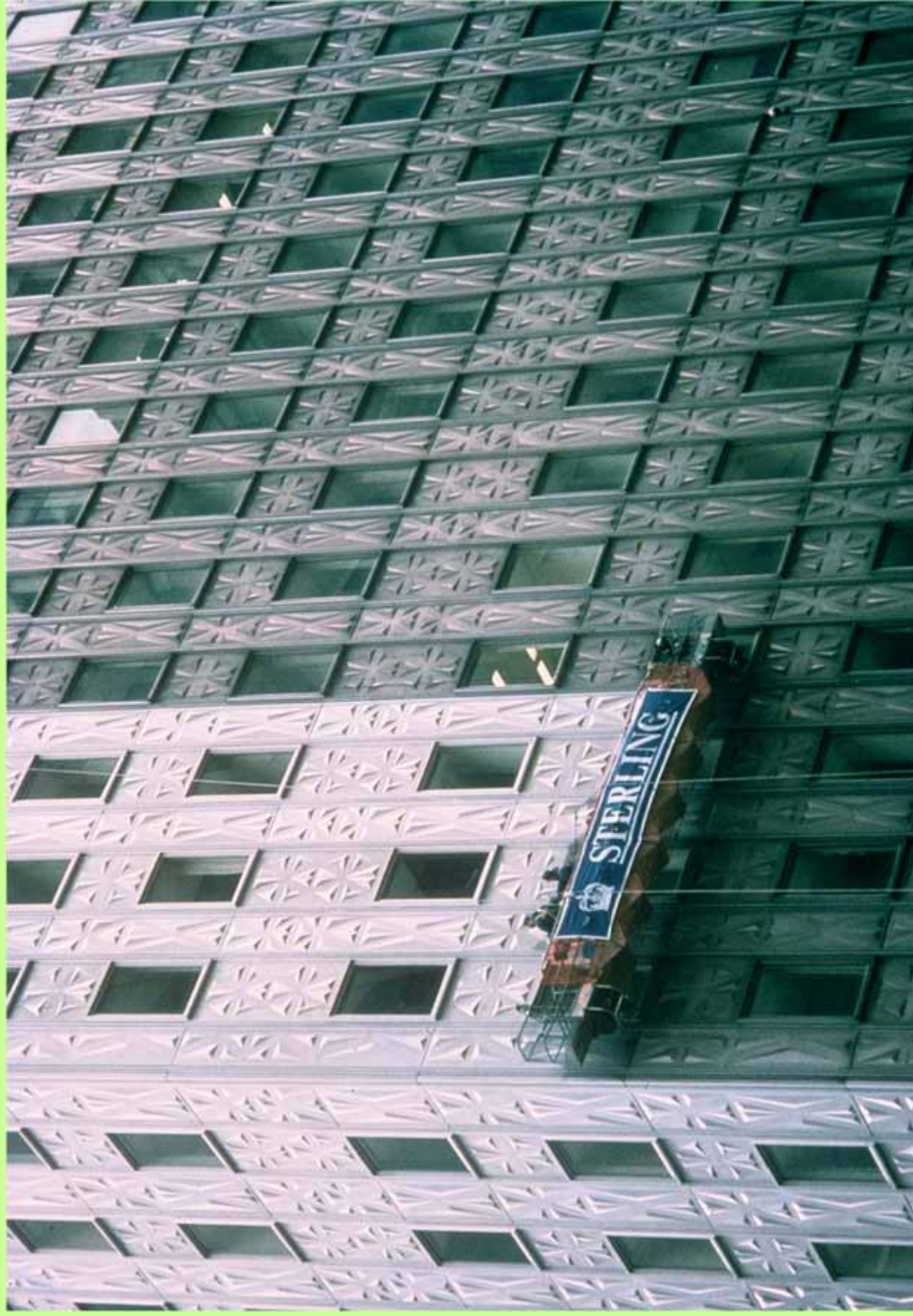
150 East 42nd Street, New York City Cleaned for the first time after 40 years of service
