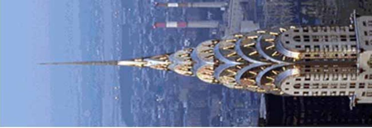
Chrysler Building 1930 First large stainless roof. Cleaned only twice.
