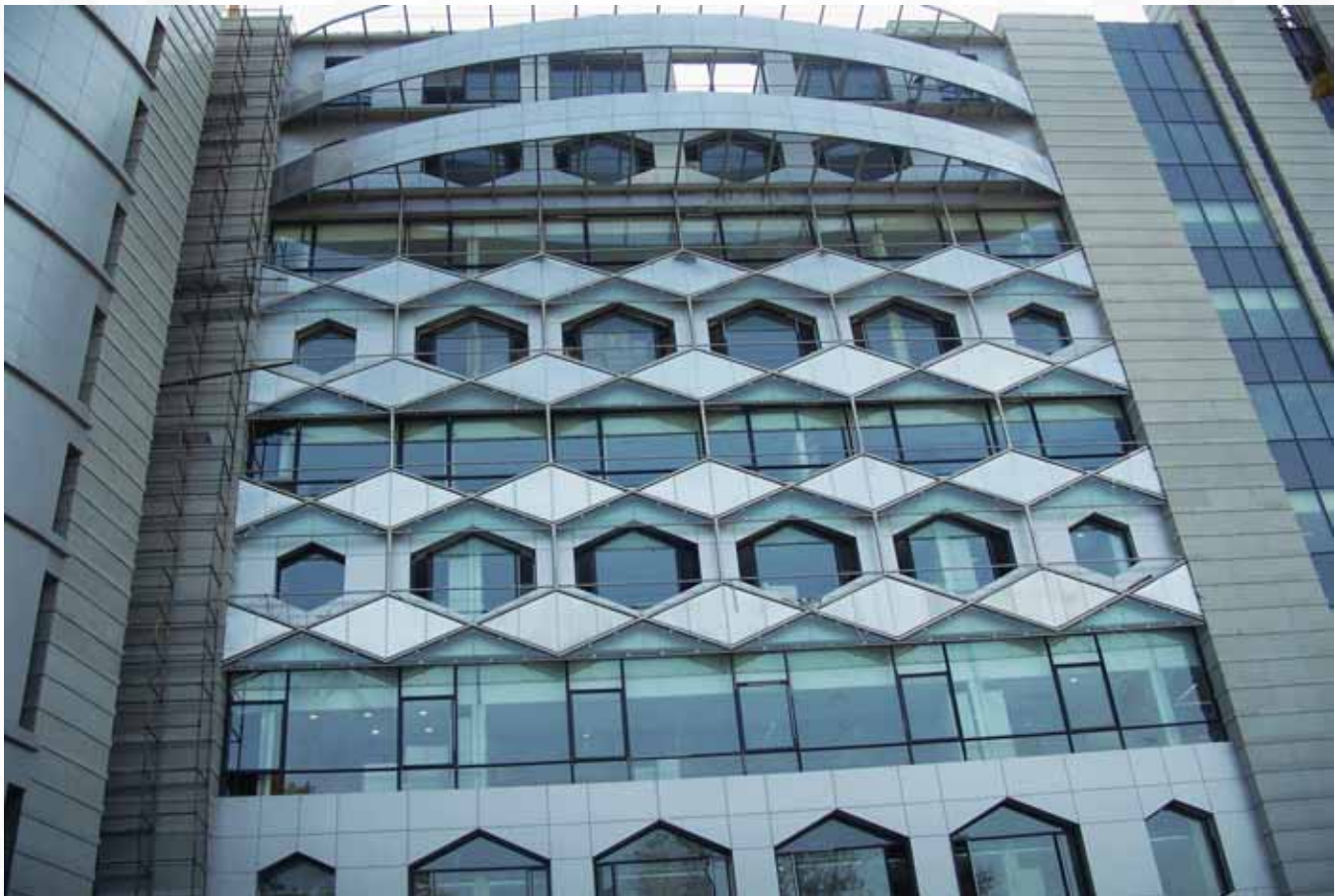
DMRC Operational Head Quarters at Barakhamba Road, New Delhi
