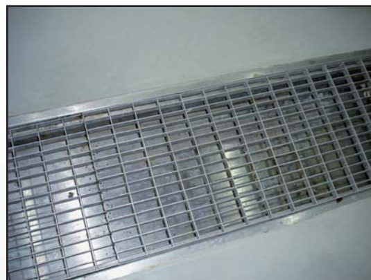
Drain with grating in stainless for corrosion-free clean floors
