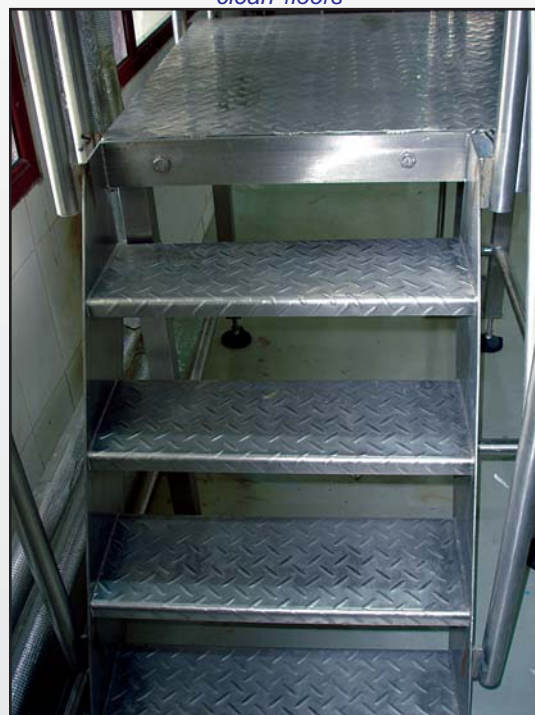
Staircases with non-skid steps of stainless steel
