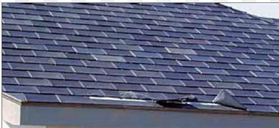
Dark gray colored stainless steel tile roof in the Bahamas. After a direct hurricane hit at 160 miles an hour (256 Kmph), this roof suffered only a minor damage as can be seen in the picture above. All of the surrounding homes lost their roofs. This is a living proof of the capability of stainless steels to resist calamities. In Japan, large stainless steel storage tanks for water have been made to withstand earth quakes to ensure water supply to the stricken people.
