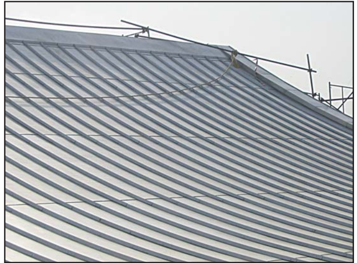
Closer view of the stainless steel roofing of the auditorium
