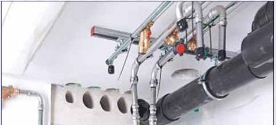
*The utmost care was taken in preparing for the assembly in the Antarctic: Openings for the drinking water installation realised with the Viega “Sanpress Inox” system made of stainless steel 1.4521. (Photo: Viega)*
