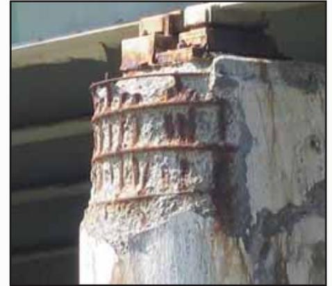
**Fig 1. Cracking and spalling of concrete due to rebar corrosion**
