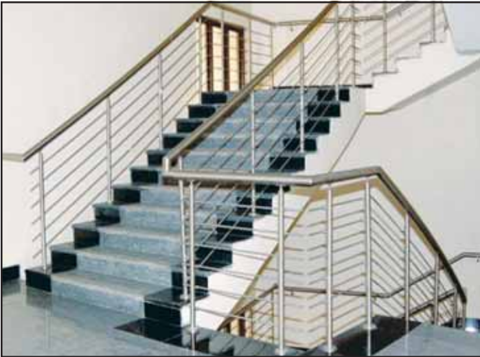
Top mounted round baluster system with horizontal members in stair case area. These 1100mm height railing system is suppose to be a high traffic area.
