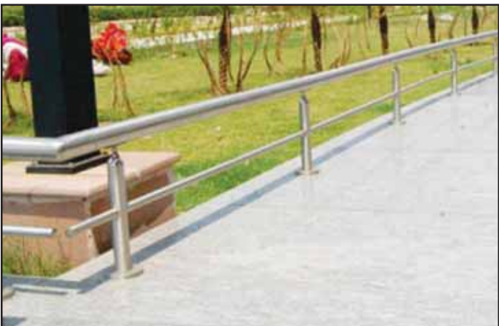
Outdoor area of campus have been adorned with these short height railing system with AISI 304 Grade Stainless Steel.
