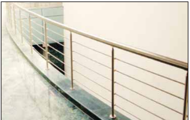
Atrium areas are beautified with 38mm dia AISI 304 Grade stainless steel top mounted round baluster system with horizontal solid
