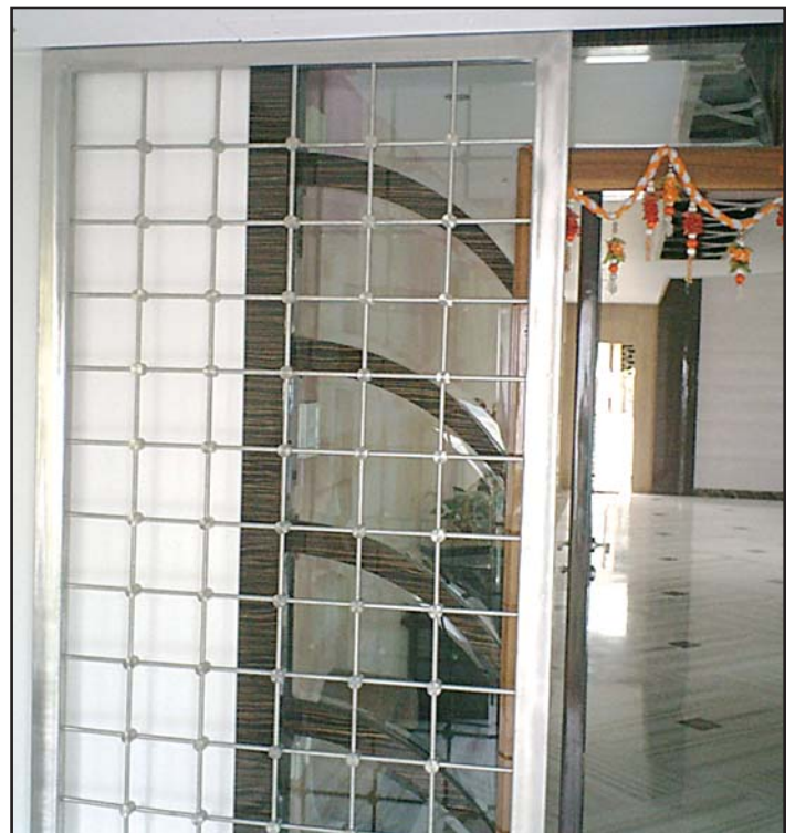
At a Kolkata home, a stainless steel sliding door, with locking arrangement, made of rectangular tubes and bars.
