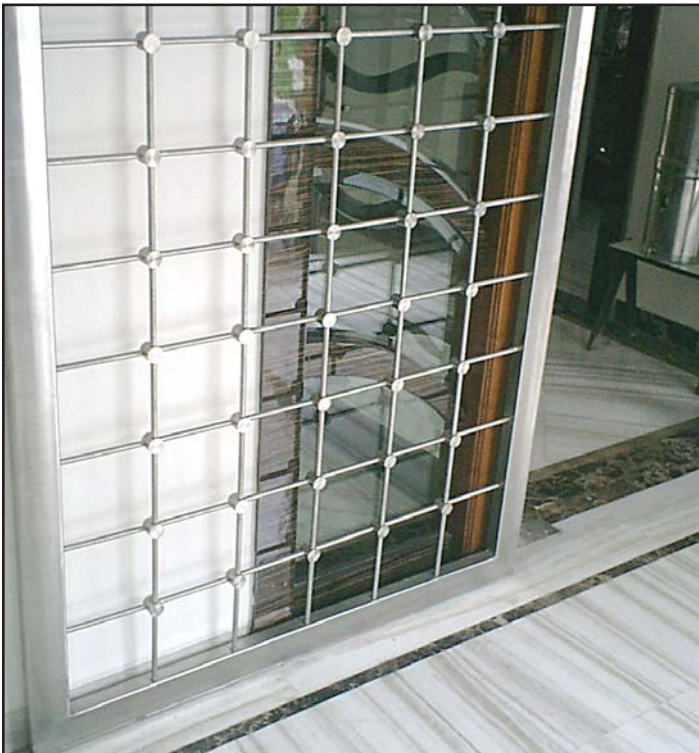
At a Kolkata home, a stainless steel sliding door, with locking arrangement, made of rectangular tubes and bars.
