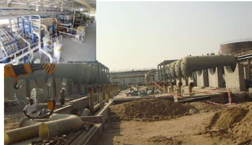
25.2 MLD seawater reverse osmosis plant at Mundra, Gujarat for the 4000 MW Ultra Mega Power Plant
