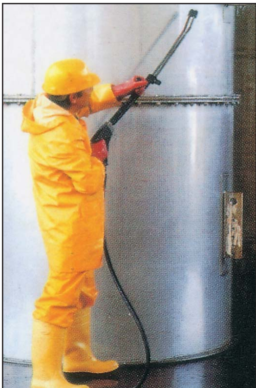
Bulk pickling of a process vessel.
