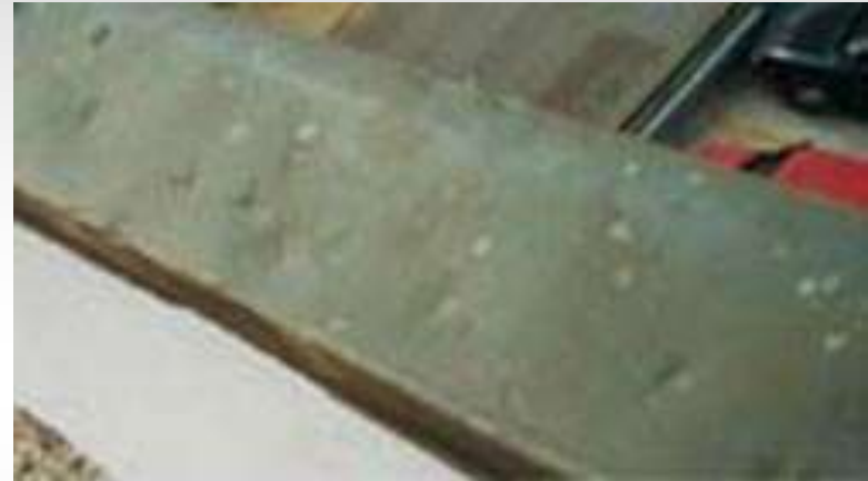
Copper hail damage
