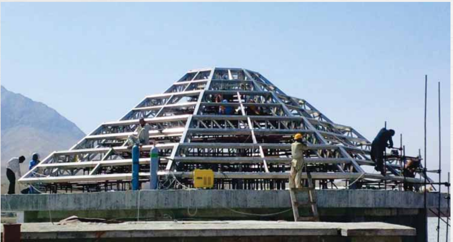
Dome of the main assembly hall under construction
