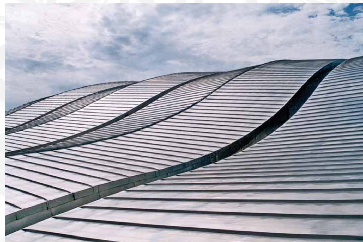
The grandstand for the Singapore Racecourse in Kranji boasts a standing seam roof comprising undulating curves achieved with Type 316 stainless steel. Photo © Erhard Pfeiffer. Photo courtesy Ewing Cole
