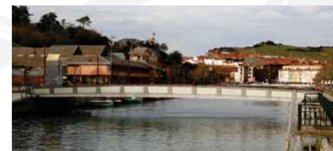
This Spanish bridge in Vilafant provides a pedestrian crossing over high-speed and traditional rail tracks.
