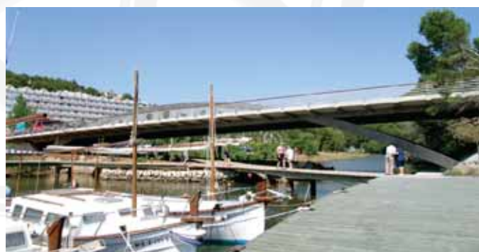
Pedelta's Cala Galdana Bridge in Menorca, Spain, uses duplex 2205 stainless steel structural components. Photo © Juan Sobrino
