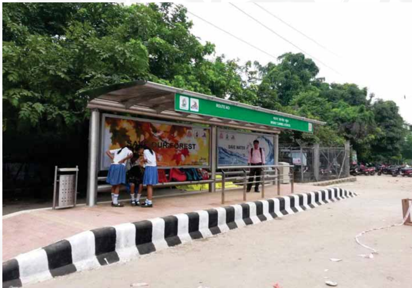
A Newly Built Stainless Steel Bus Queue Shelter at Patna
