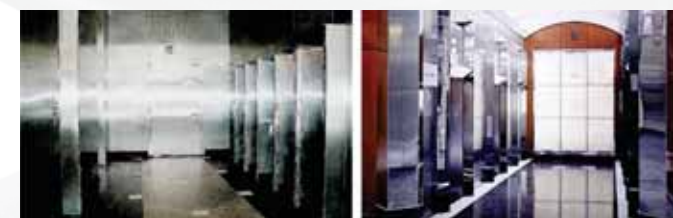
After 50 years of oil and wax 'cleaning,' the stainless steel in this lobby was dark from dirt and grime accumulation and had some scratching (left). The panels were taken down, cleaned with dishwashing detergent, refinished
