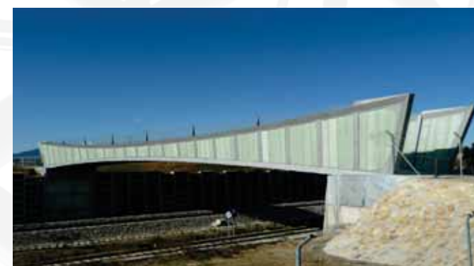
Image 1 of 3 - This bridge, for the small Basque city of Zumaia, needed to withstand the maritime climate, achieve a long service life, and be lightweight. Duplex stainless steel fit the bill. Photo © Ricardo Ferraz
