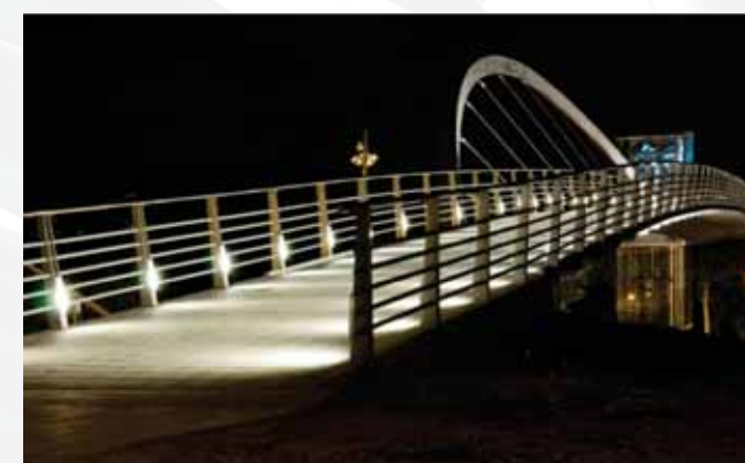
Spain's San Fruitos Bridge (2009) employs duplex 2304 stainless steel to cross a highway. Photo © Jasper Hermen
