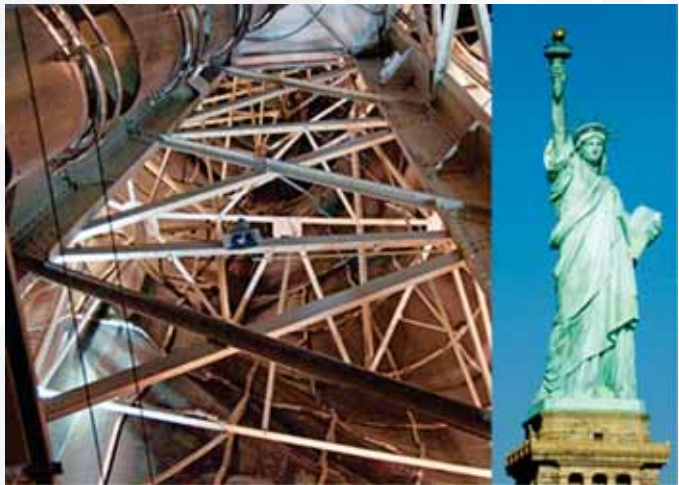
The 1986 restoration of the Statue of Liberty used duplex stainless steel to replace much of the original iron support framing. Photo © Mike Renlund and Erik Cleves Kristensen (inset)
