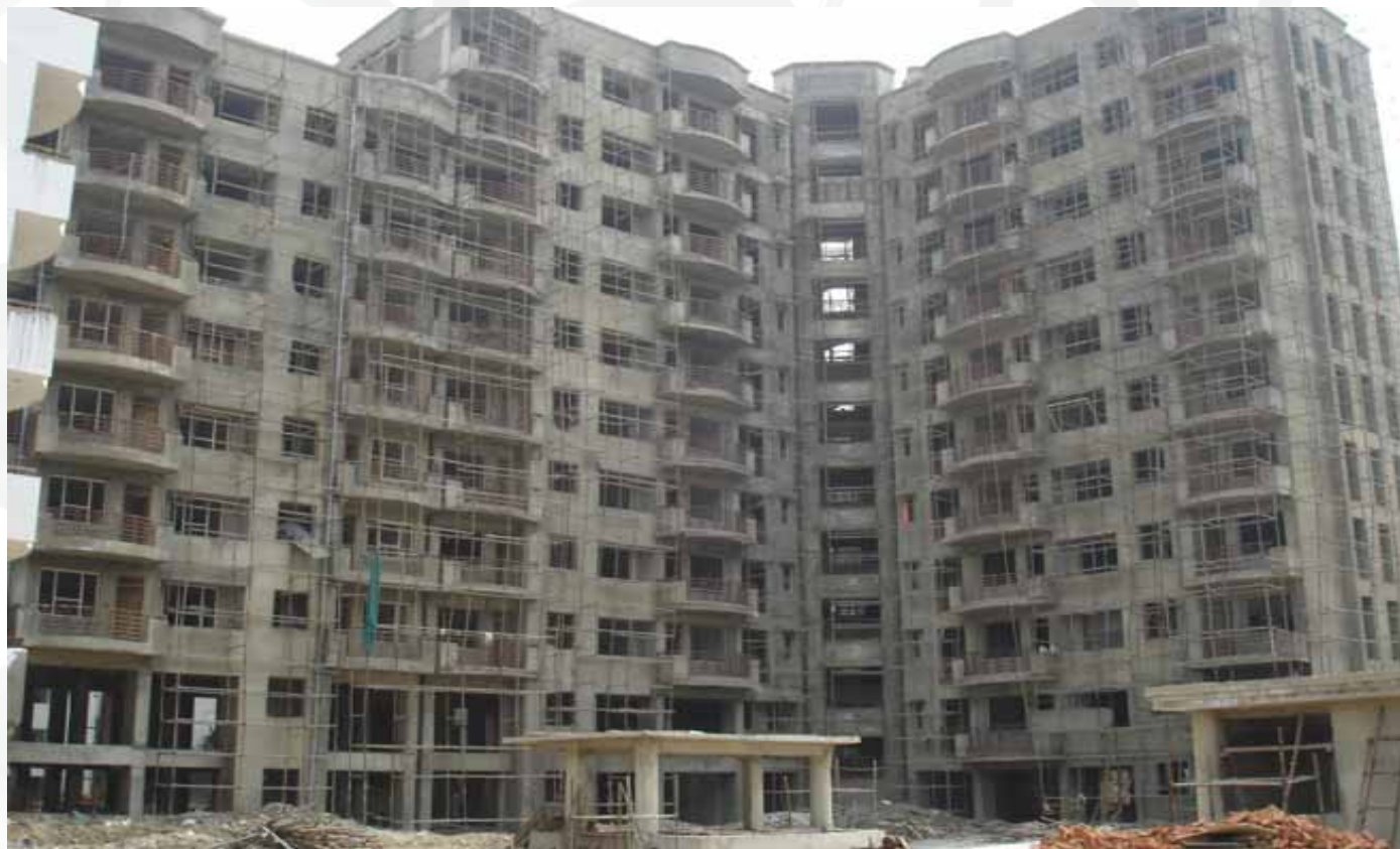
*PIC* - Front of whole Building, Pipe fitted to wall, Press fitting tool old,
