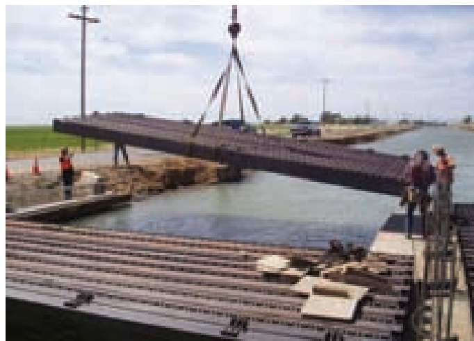
ASTM A1010 Stainless Steel Bridge Under installation- USA
