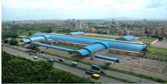
Koparkhairane Railway Station in Navi Mumbai. 10,000 sq.m resin-coated curved roofing
