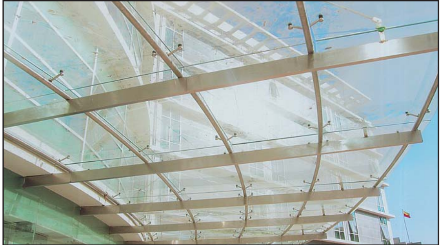
Carbon steel I-beams clad with stainless steel sheets
