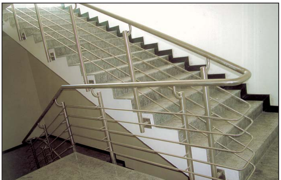
Stainless steel staircase handrails
