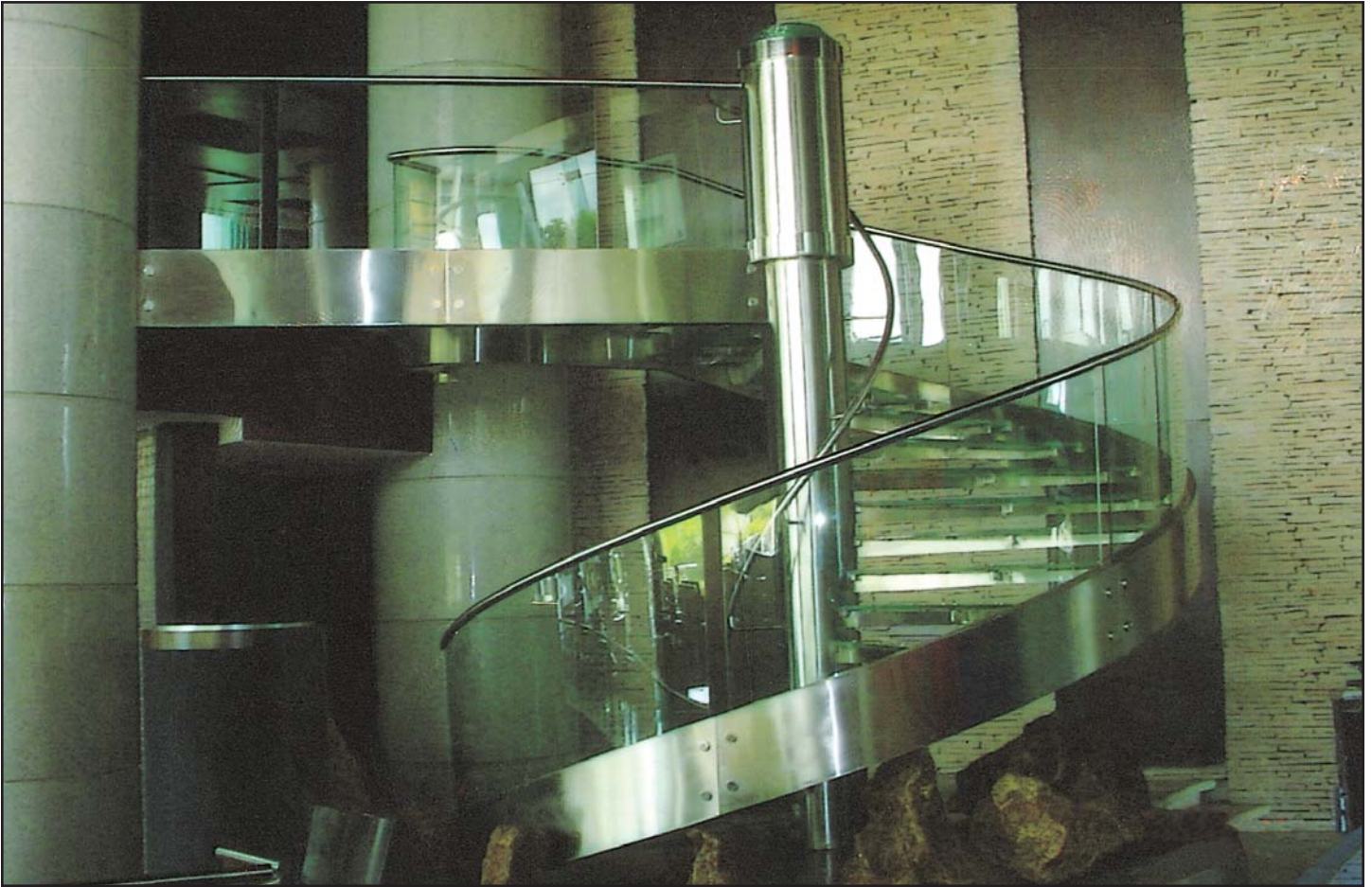
Spiral staircase at Hyatt, Mumbai. AISI 316 stainless steel, 1.6 mm stringer, 40 mm dia handrails. Toughened glass has been used as the balustrade and the steps are made of laminated glass. The central hollow column is made of stainless steel.
