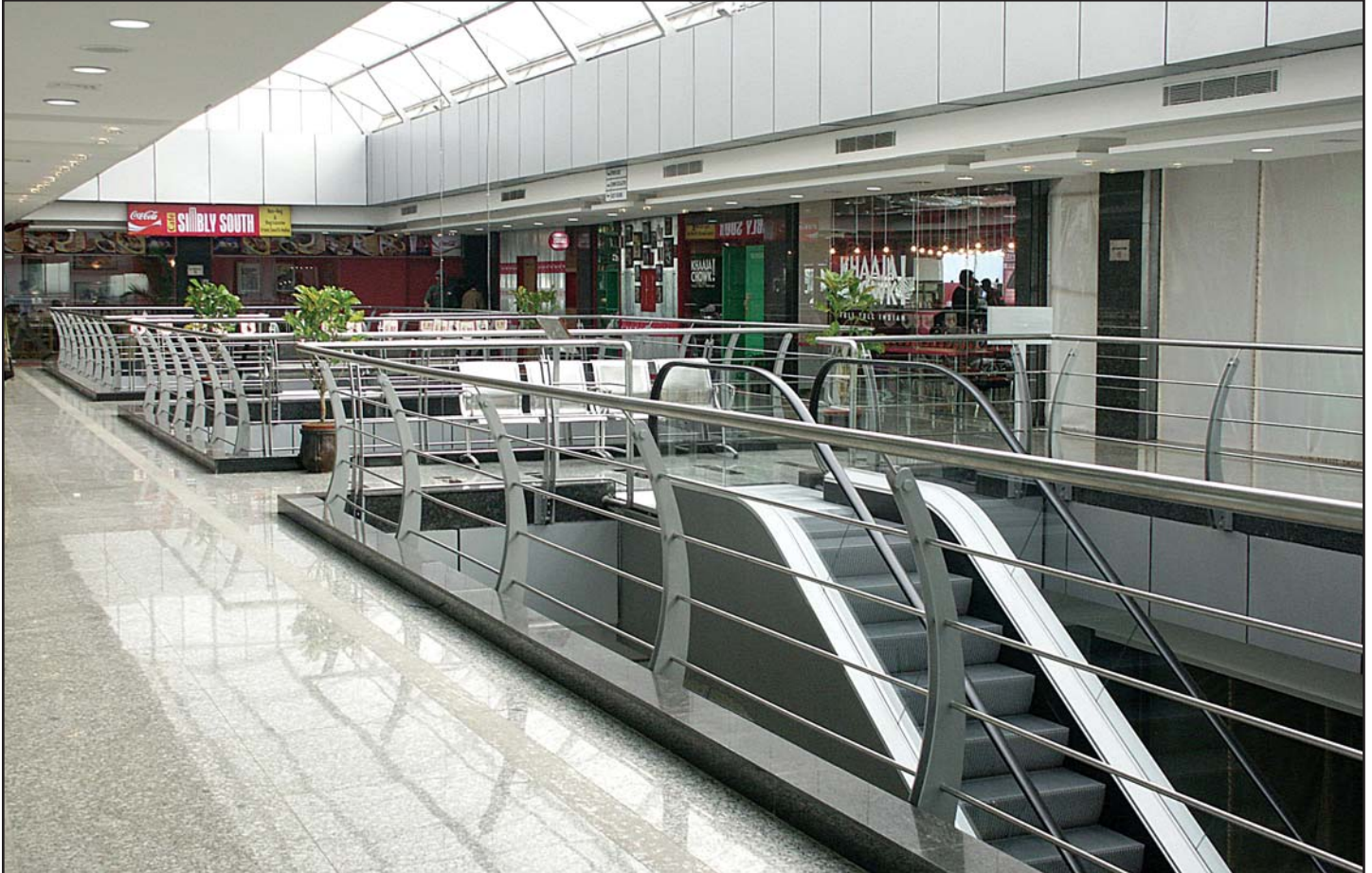
The Plaza Mall, Mehrauli Gurgaon Road, near IFFCO Chowk, Gurgaon - 1,800 running metres of handrails of AISI 304 stainless steel in Brush Finish.
