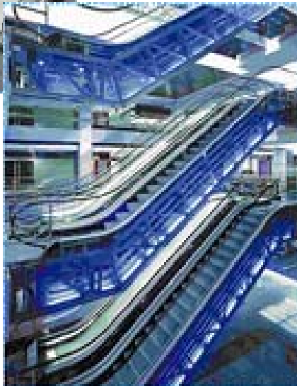
Escalators in a shopping mall
