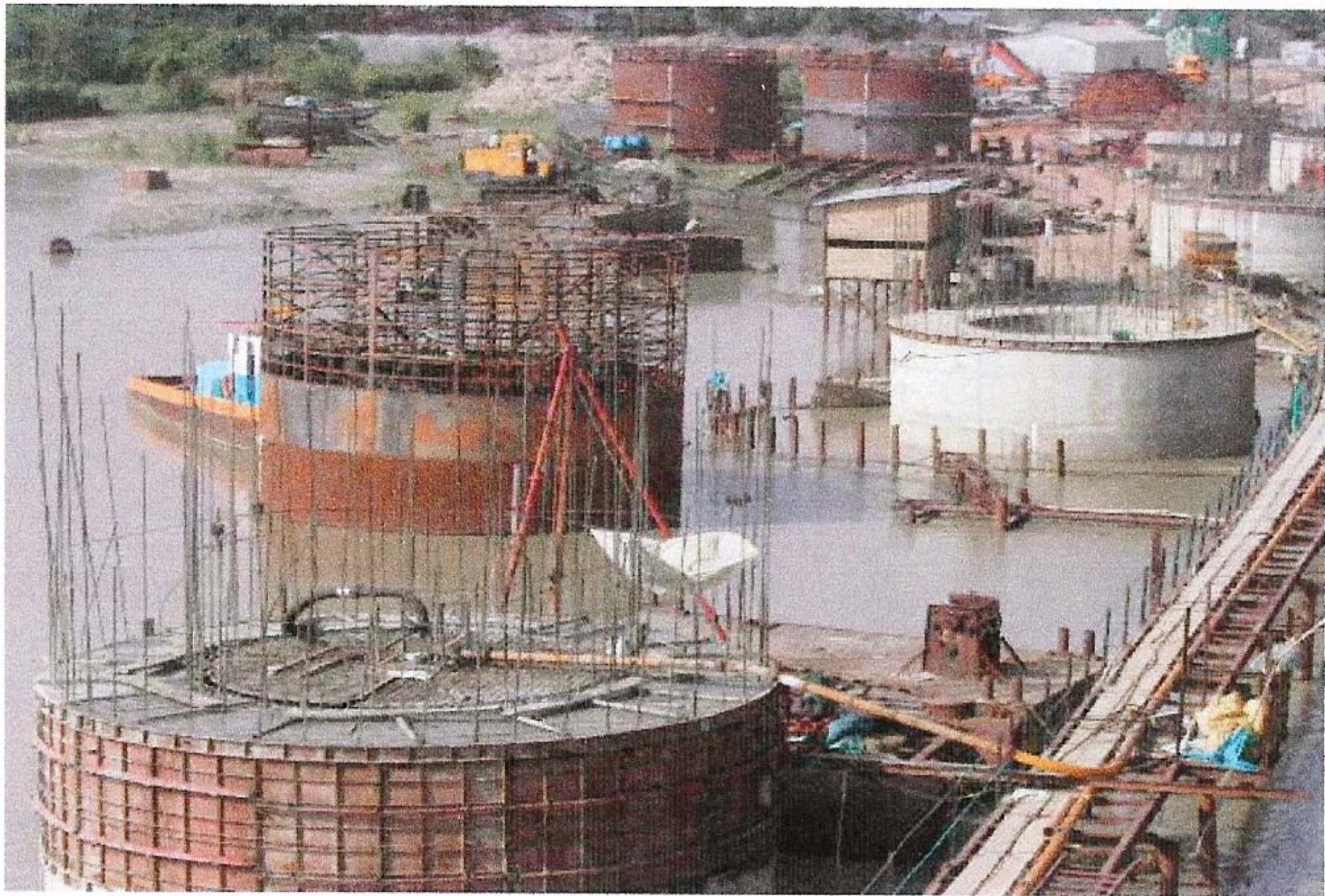
Rupnarayan Bridge at km 73.486
