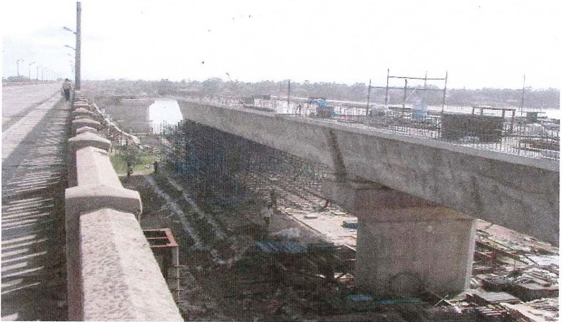
Rupnarayan Bridge at km 73.486
