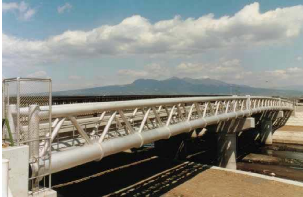
Lightweight Bridge to carry drinking water in Tokyo.
