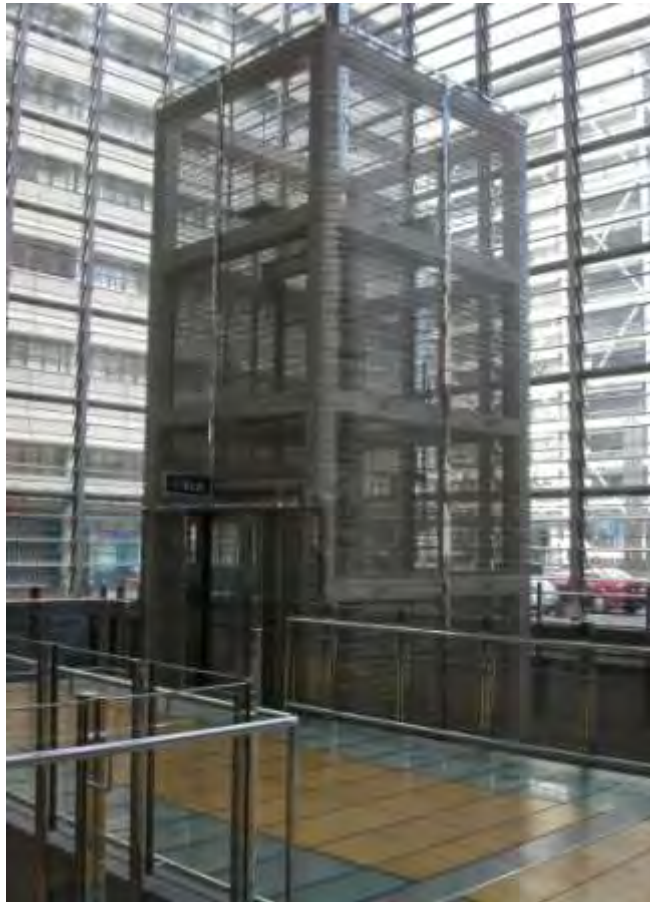
Lift tower covered in Type 316 stainless steel mesh
