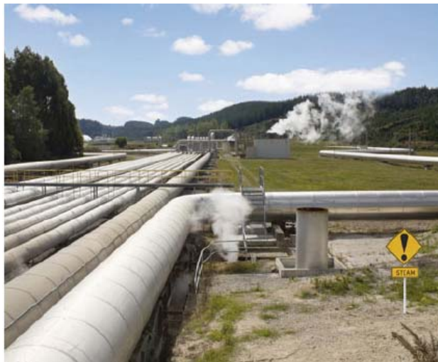
Geothermal plant (Ren21)
