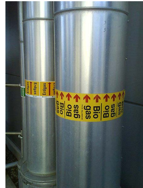
Pipes carrying biogas, natural gas and condensate (Wikipedia)
