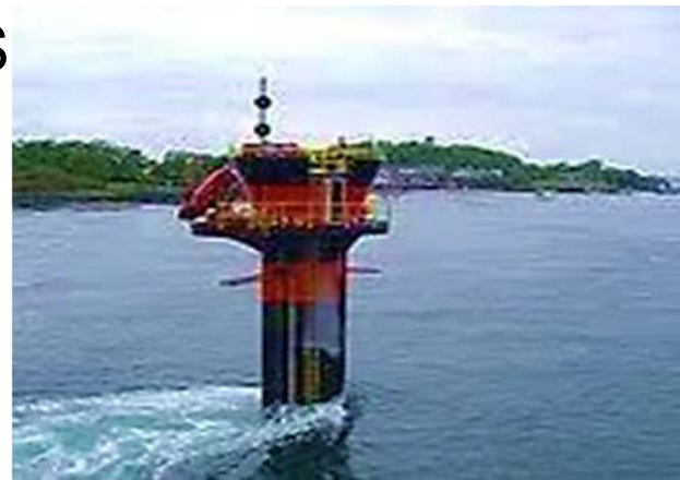
First commercial grid-connected tidal stream generator, Strangford Loch, U.K.
