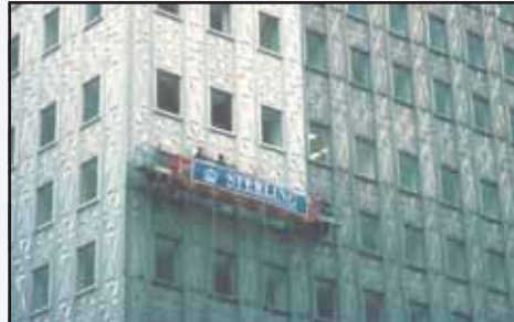
Socony-Mobil being cleaned.
