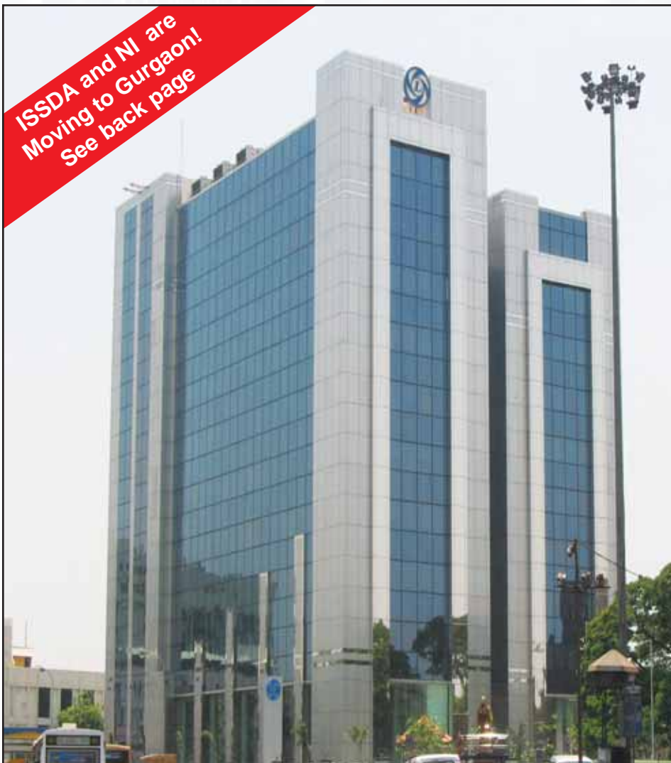
The Ashok Leyland HQ Enveloped in Stainless Steel Composite Panels & Glass
