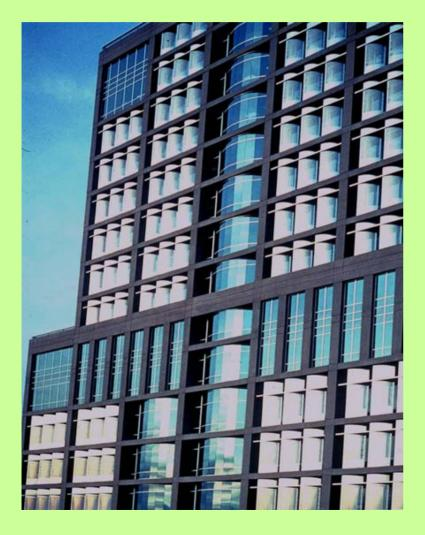
**PHOENIX CITY HALL** Perforated, polished stainless steel window shades; US\$285,000 one time capital savings in installing A/c equipment; US\$200,000 annual air conditioning savings in electricity
